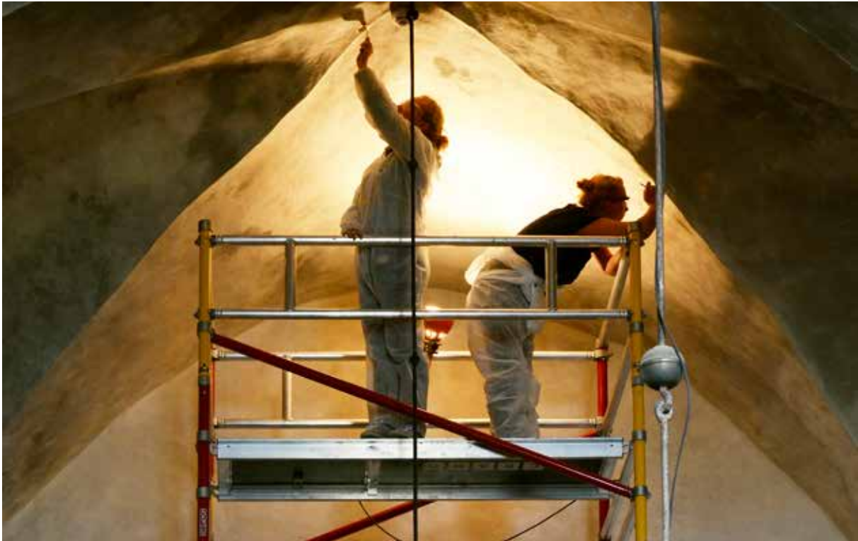
Photo 20. Summer internship for EAA Department of Cultural Heritage and Conservation students: investigations of the finishing layer in Haljala Church. Photo by Peeter Säre
