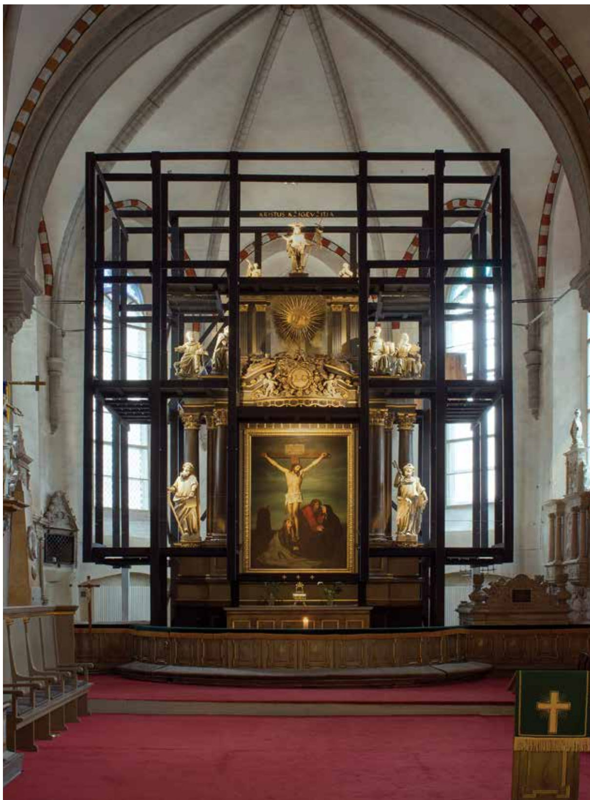
Photo 18. A wood structure made by students of the EAA's Departments of Interior Architecture, Graphic Design and Cultural Heritage. It frames the Tallinn Cathedral's Baroque altar permitting researchers and visitors led by a guide to climb to a height of almost 10 metres. Supervisors: Hilikka Hiiop (EAA Department of Cultural Heritage and Conservation), Hannes Praks (EAA Department of Interior Architecture), Tiina-Mall Kreem (Art Museum of Estonia) Kristjan Holm (EAA Department of Interior Architecture), Juhan Kilumets (Rändmeister OÜ) Students: Johanna Sepp, Ardo Hiiuväin, Elin-Harriet Helemae, Ellen Sepp, Kaia Tungal, Martin Siplane, Maria Kesküla, Tiina Sakernmaa, Taavi Tiidor, Aimur Takk, 2016. Photo by Peeter Säre
